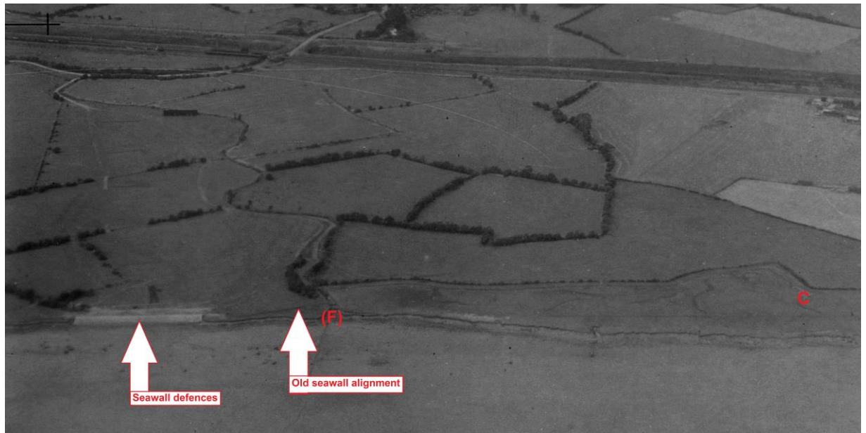
Photograph B: showing 1951 Seawall construction
